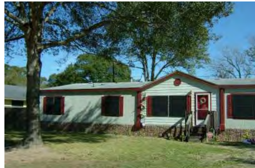
Example of a HUD Code manufactured home
