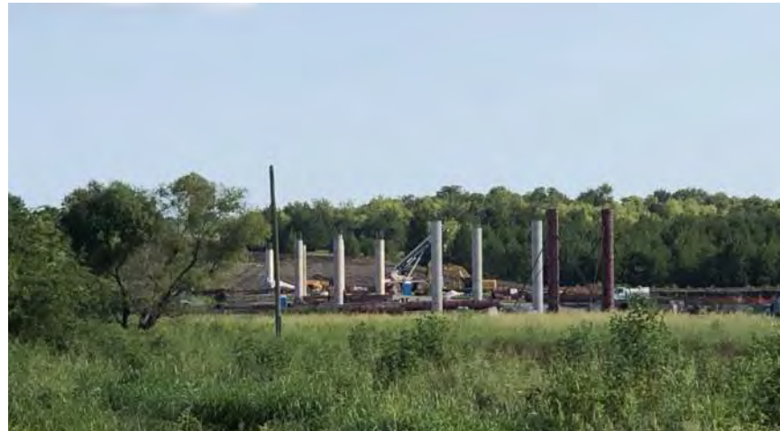
Construction of the SH 34 Bridge in August 2021
