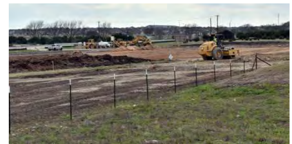
Limit clearing and grading near the Lake Ralph Hall
