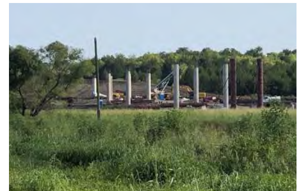
Construction of the SH 34 Bridge in August 2021
