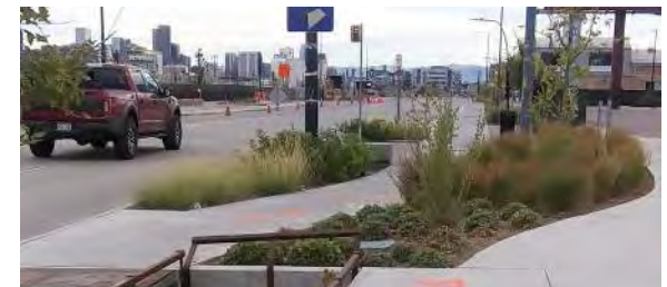
Encourage low impact development, such as bioretention basins, to remove contaminants from stormwater runoff
