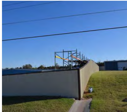
Good example of contractor yard screening
